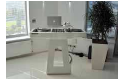
Because the DJ console is integrated into the control system, it's easy to pipe music into every room during a party.
