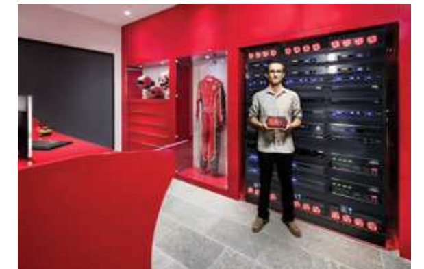
Project Installation by Lifetronic
