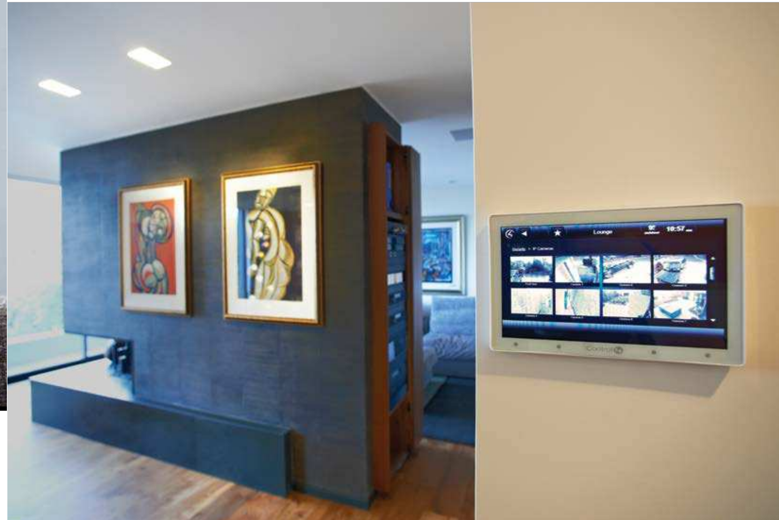
A perfectly positioned touch screen makes it easy to monitor the whole home from one location, and control the fireplace, adjust the lights, and so on.
